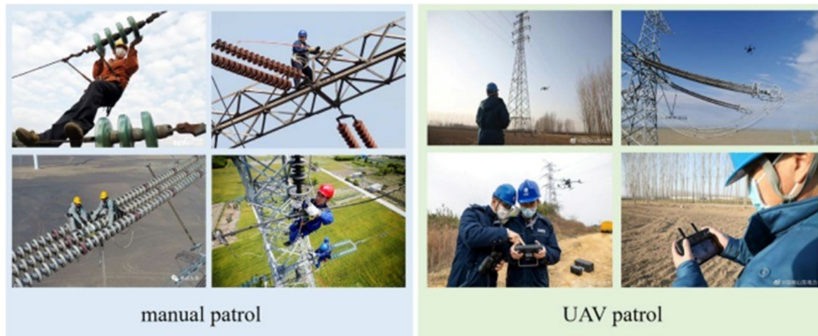
Figure 1: The overhead electrical line inspection procedure.
