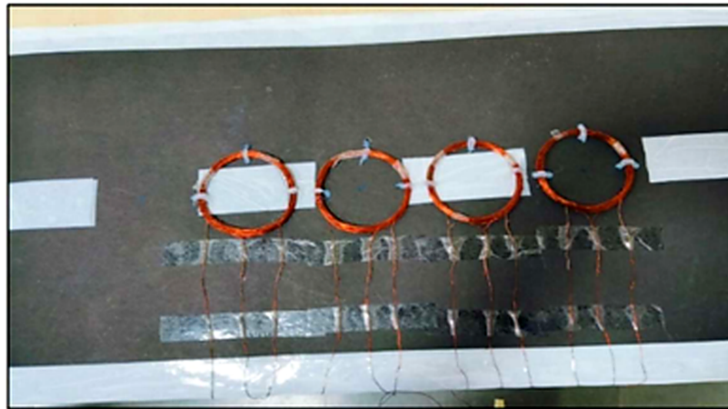
Figure 8: Installation of transmitter coil on road.
